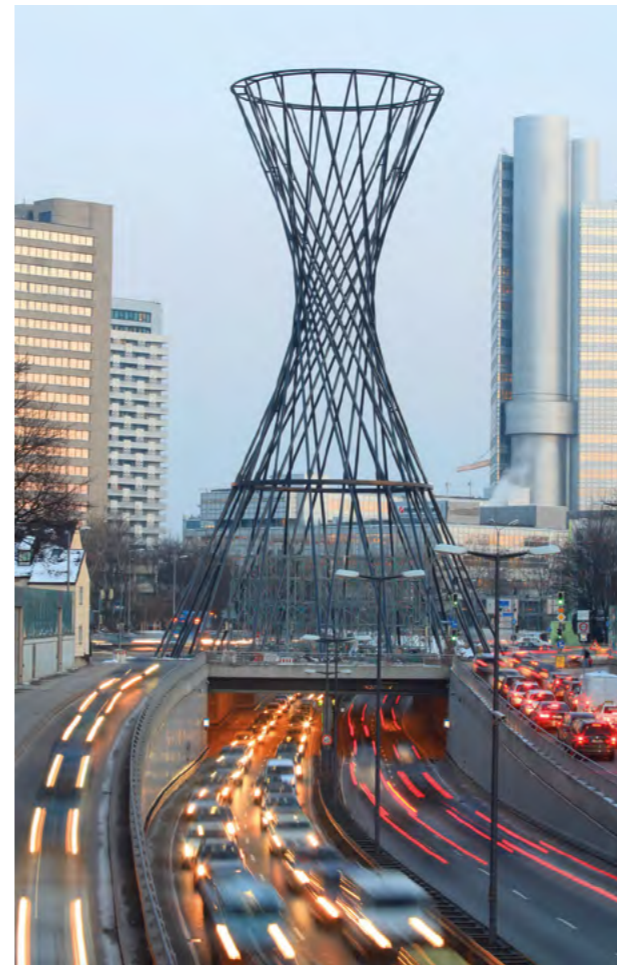
f.i.t.r. ■ Mae West Sculpture in Munich (Effnerplatz) produced with Biresin® CR84. ■ Segment of a 40 m pipe used for the Mae West sculpture.
